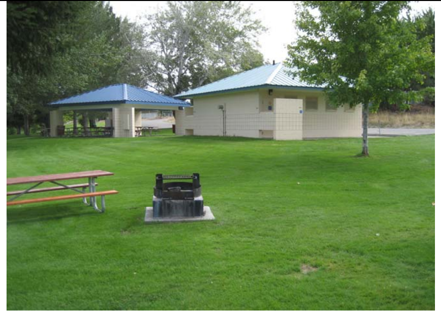
Picnic shelter & restroom
