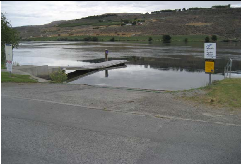
Boat launch ramp & handling dock
