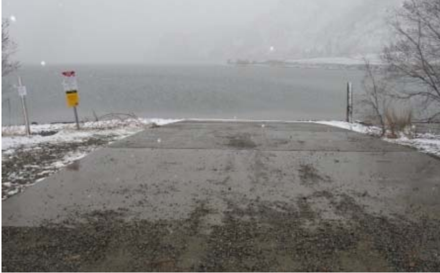
Concrete boat launch ramp (two lanes)
