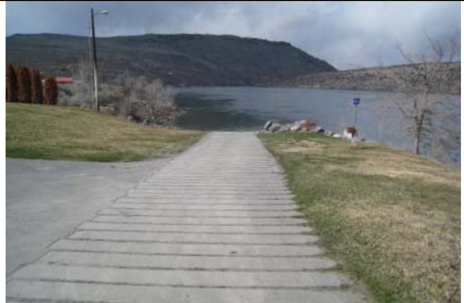
Concrete boat launch ramp (one lane)
