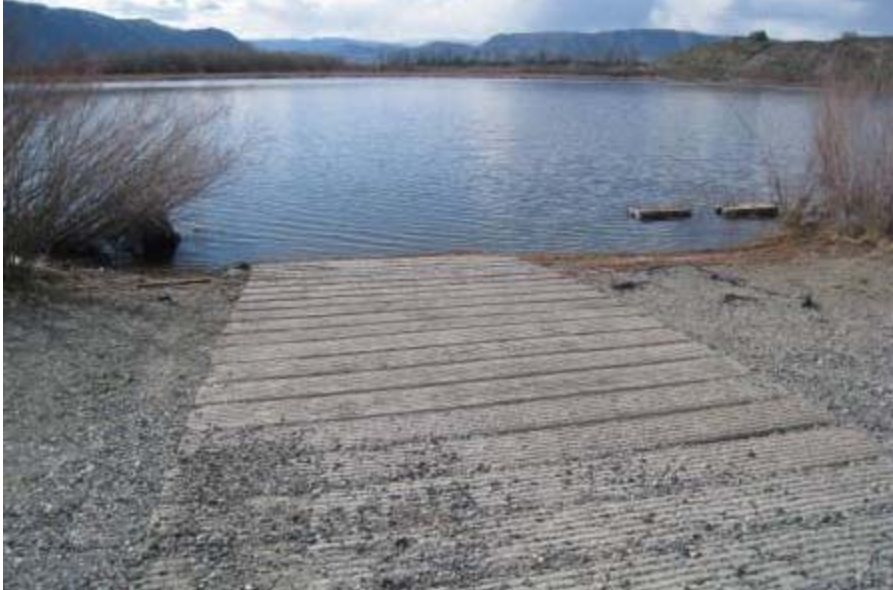
Concrete boat launch ramp (one lane)
