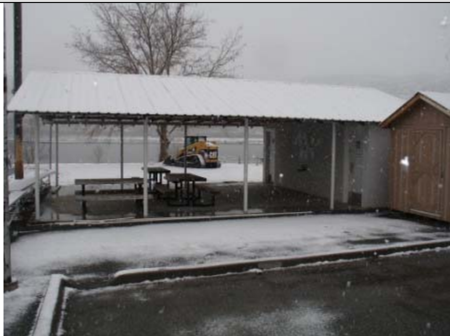
Paved parking area, picnic shelter & restroom unit
