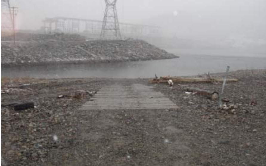
Concrete boat launch ramp (one lane)
