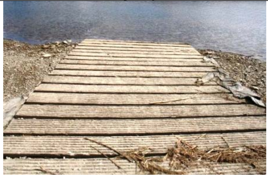
Concrete boat launch ramp (one lane)
