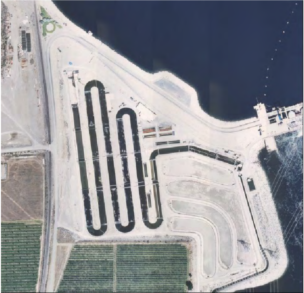
Figure 3.0-1 Aerial image of the Wells Hatchery.
