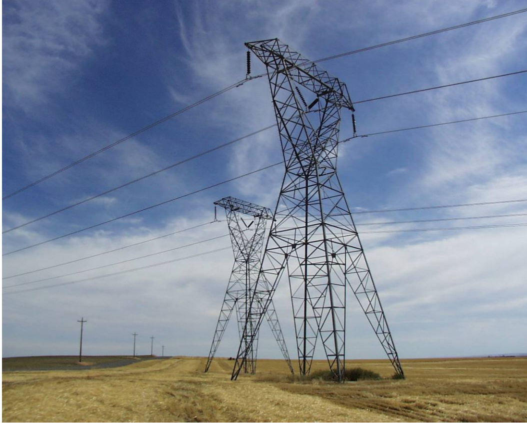
Figure 2.6-1 Wells Project transmission lines.
