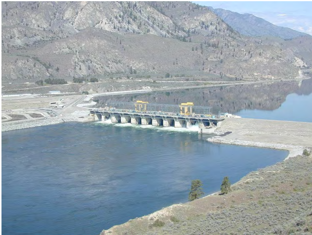
Figure 1.0-1 Wells Dam looking to the northwest.
