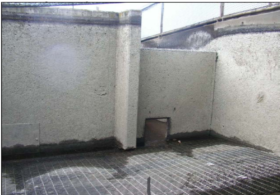
Figure 9. Floor diffuser grating and submerged orifice at the dewatered John Day Dam fishway (Richards 2007).
