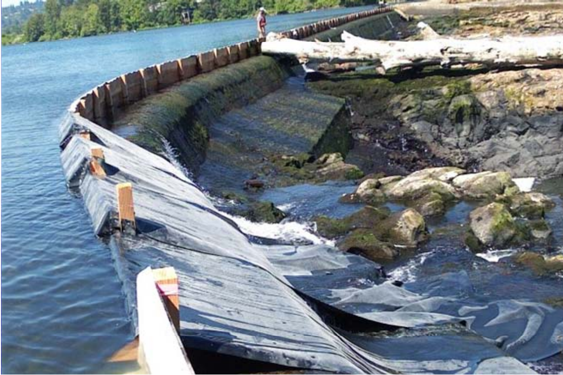
Figure 11. Lamprey passage ramps installed at Willamette Falls after flashboard installation (CRITFC 2004).
