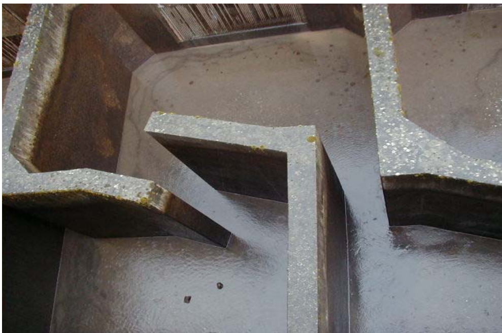
Figure 8.. Serpentine weir section at Bonneville Oregon Shore fishway (Moser et al. 2004).
