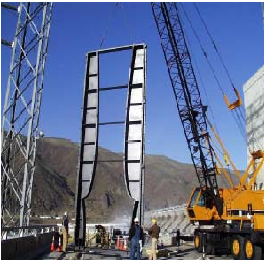
Figure 12. Slotted “key hole” fish ladder entrance installed at Priest Rapids Dam (Lauver 2006).
