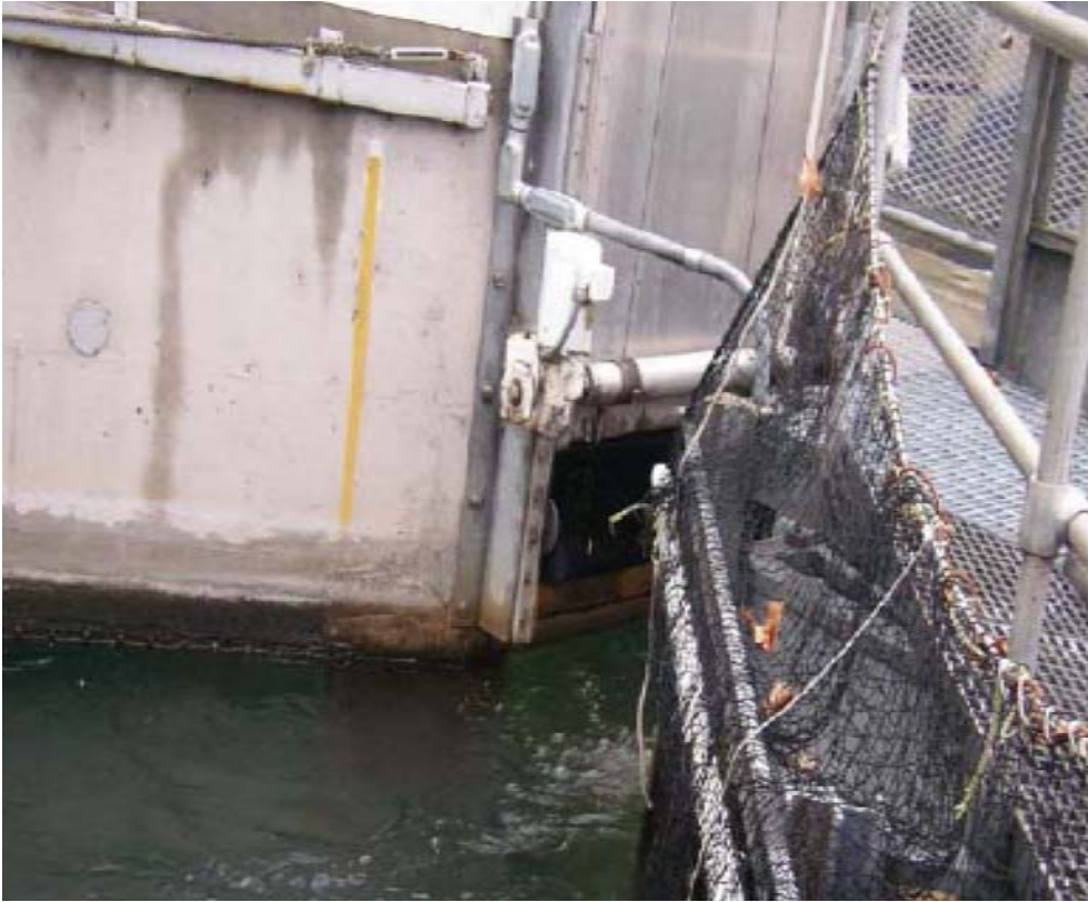
Figure 7. Counting station at the John Day Dam fishway. Note the picketed lead on the right side of the picture below the netting (Richards 2007).
