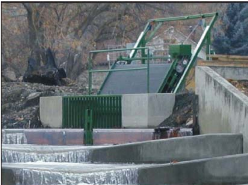
Figure 23. Traveling belt screen (BOR 2003b).
