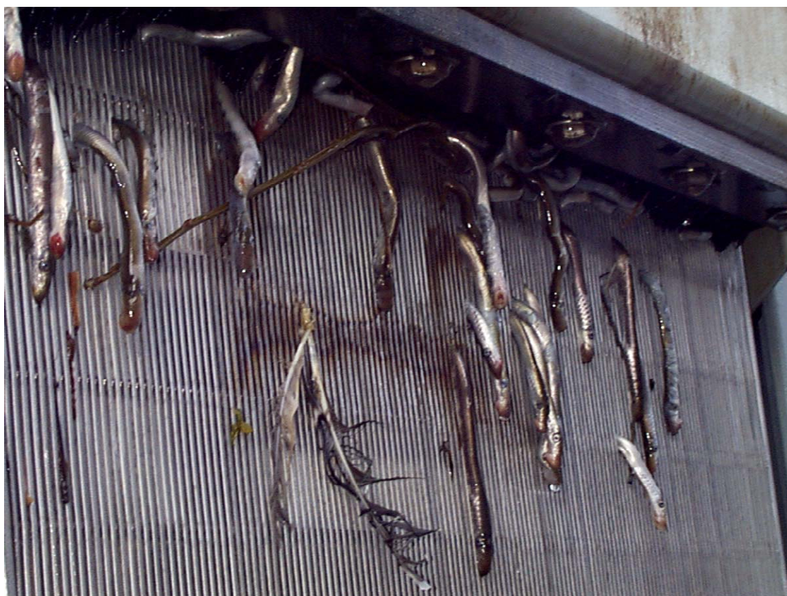
Figure 20. Impingement of juvenile lamprey on John Day extended length bar screen (Starke and Dalen 1998).
