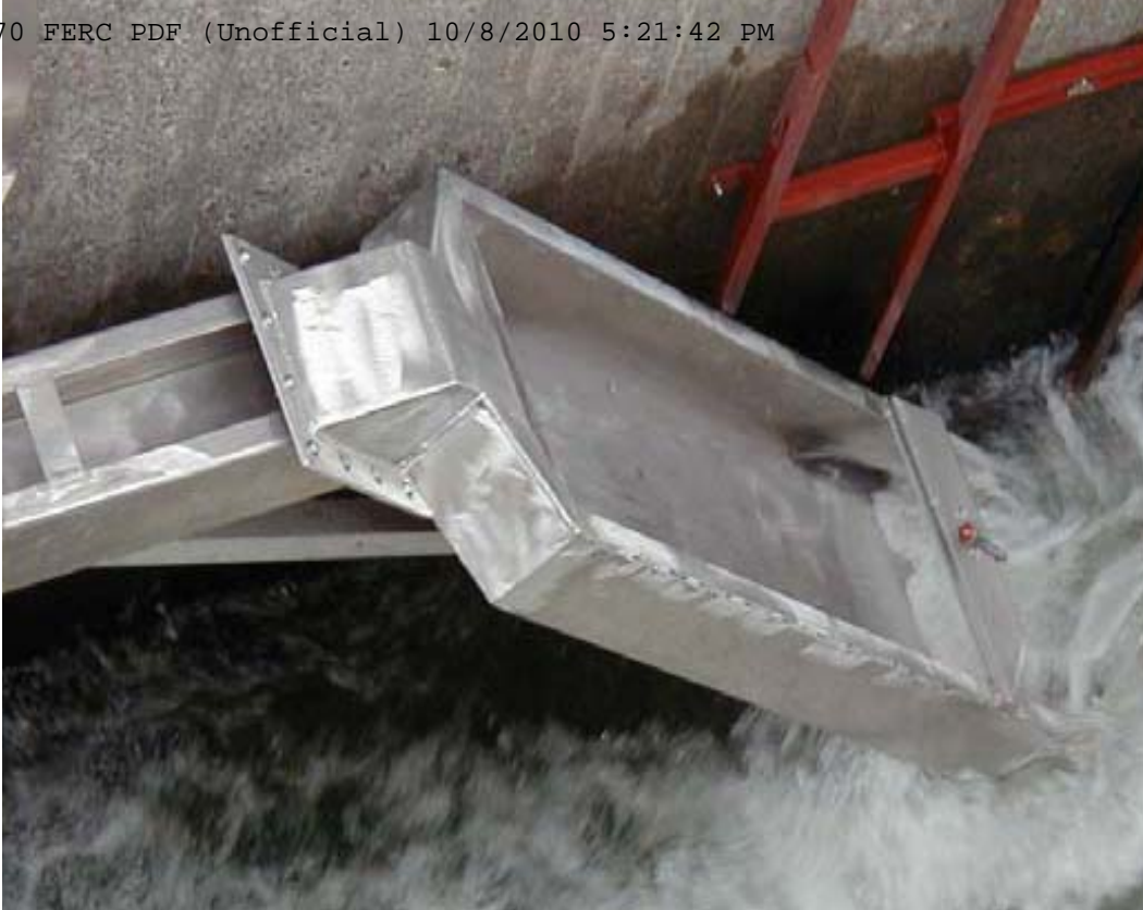
Figure 10. LPS structure at the Bonneville Dam Oregon Shore fishway. A lamprey passing upstream can be seen at the upper portion of the bottom of the structure (Moser et al. 2004).
