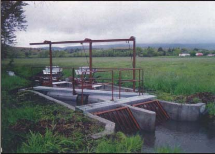
Figure 22. Drum Screen at irrigation diversion (BOR 2003b).
