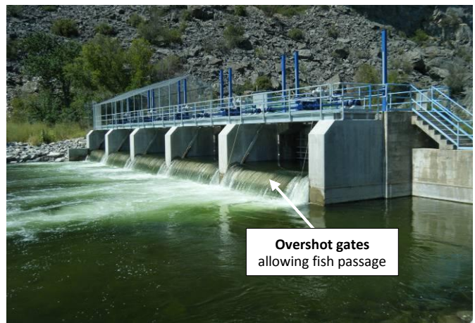
McIntyre Dam Before and After the Modifications
