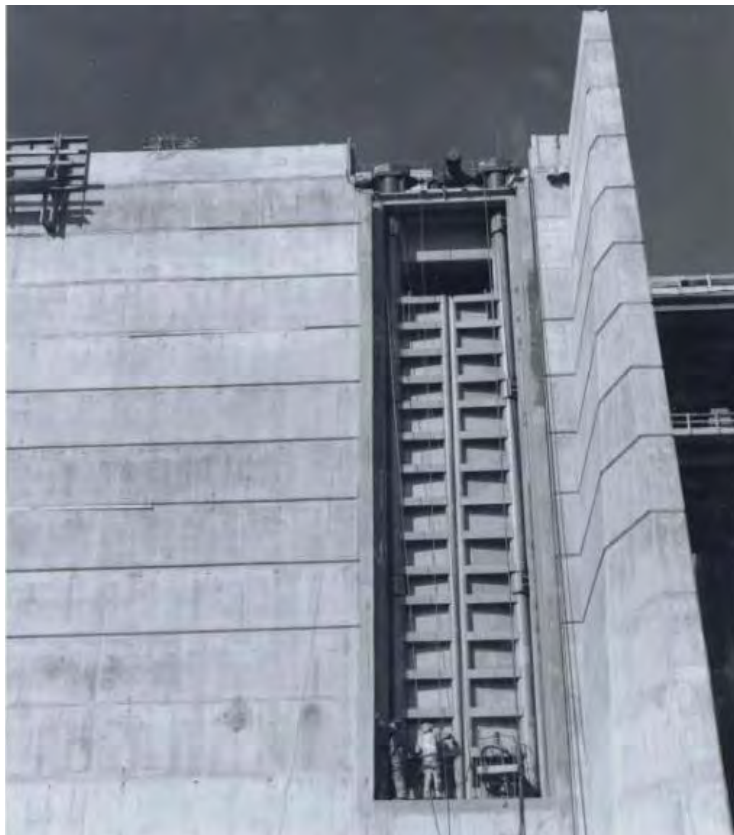
Photo 2: Looking upstream at the de-watered West fishway entrance during maintenance. In this photo the two gates are closed. (Archival Photo from Douglas PUD)
