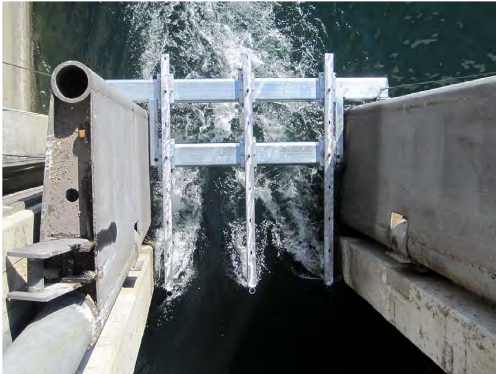
Photo 3: Looking down on the ADV trolley shown inserted in the bulkhead gate slots. (This photo was taken by Jacobs Engineering during the trolley testing in Feb 2011)
